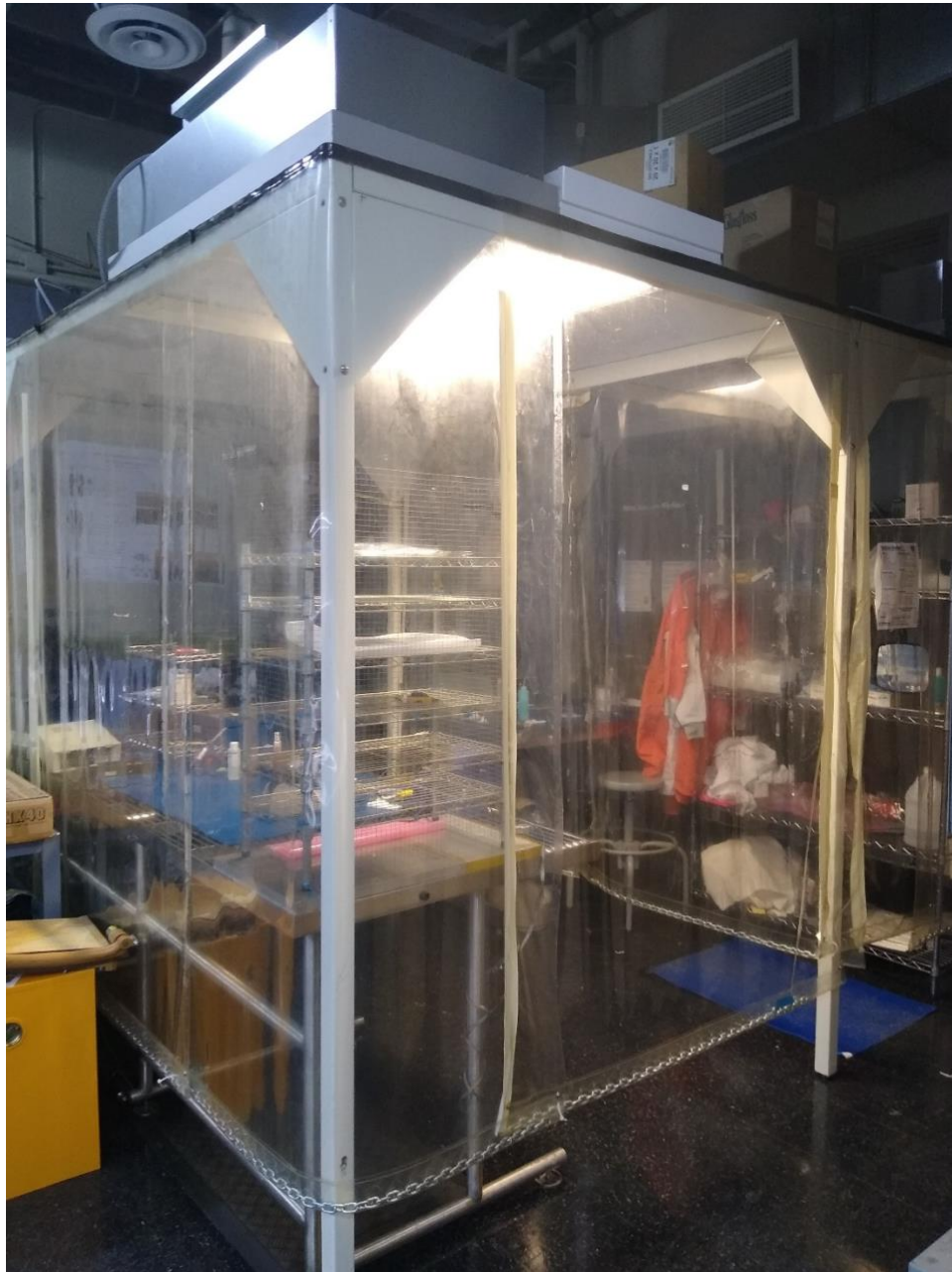
Figure 4. Class 10,000 clean room
