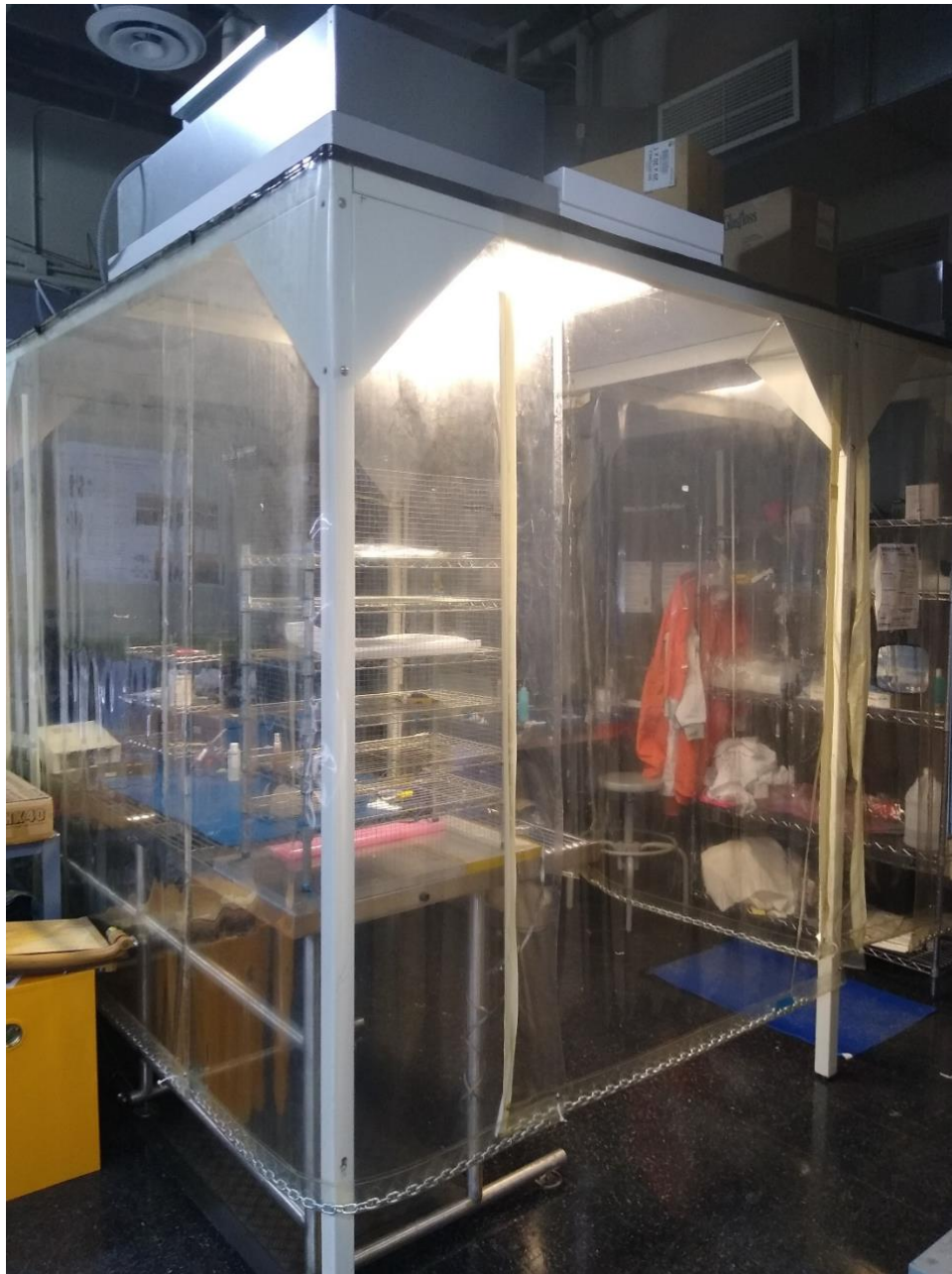
Figure 4. Class 10,000 clean room
